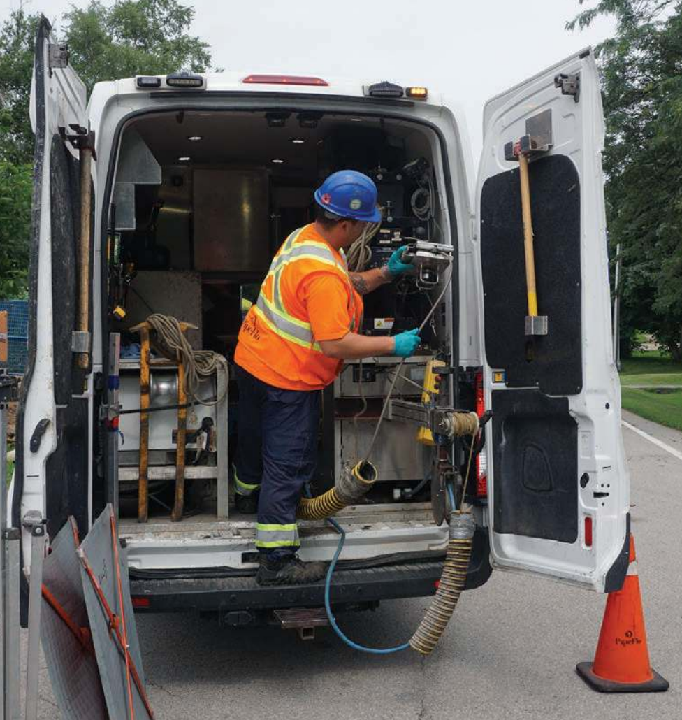
▲ Roberto Larenjeiro sets up for an inspection job with a CUES inspection system.
